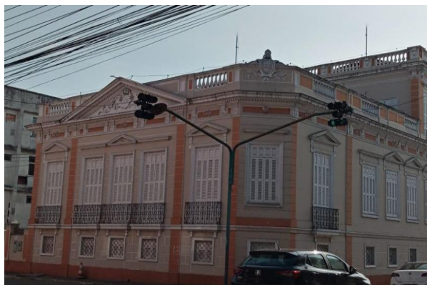
Figura 42 - Vista diagonal do Palacete Nery.
